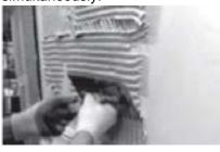
On the section of the wall, where it is supposed to install the panels, apply gypsum filling putty "Pufas" (Full + Finish)
